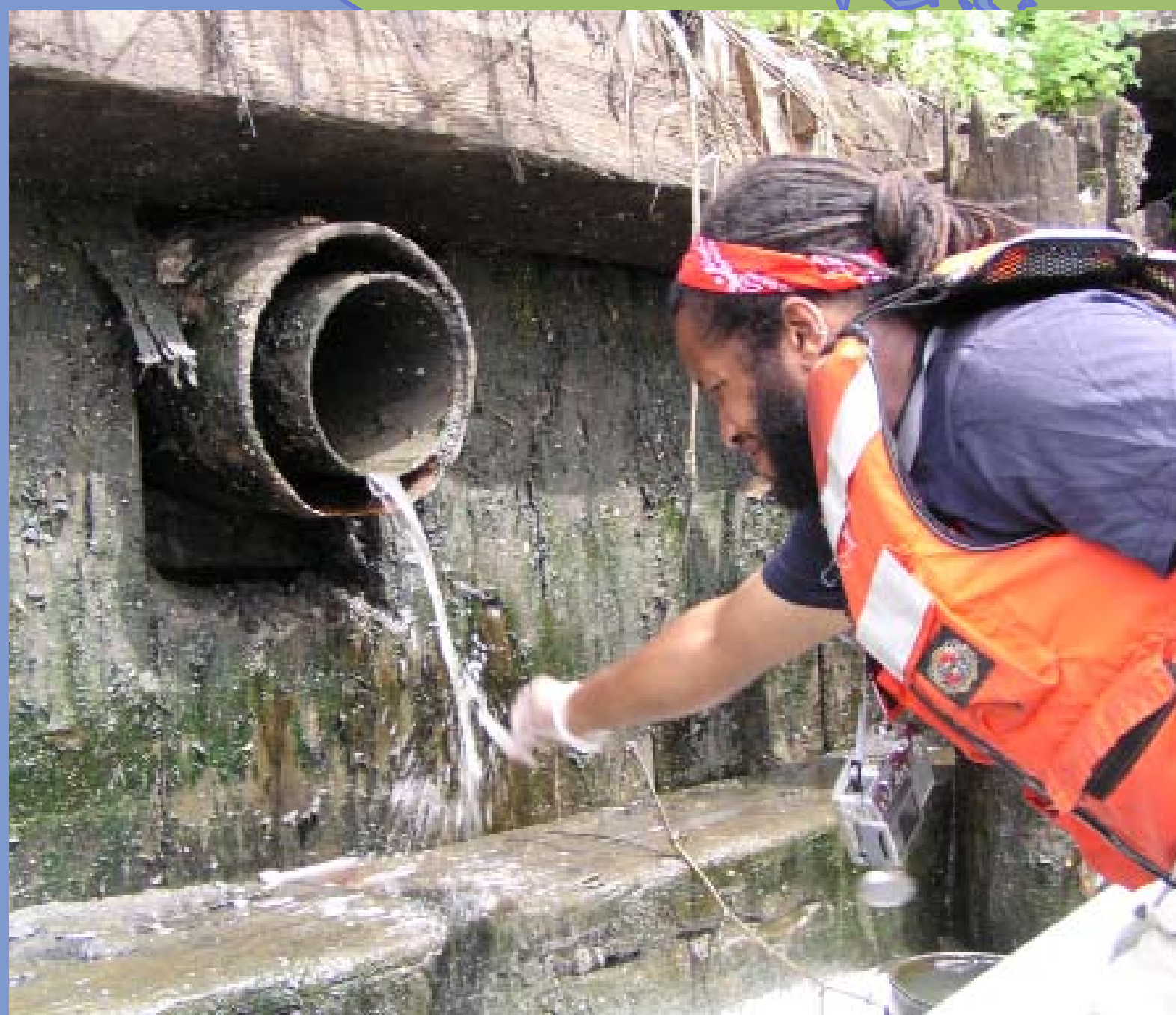
NEWTOWN CREEK OUTFLOW PIPE. PHOTO COURTESY OF RIVERKEEPER
